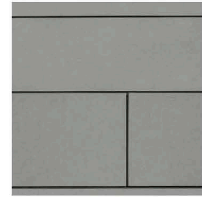
High-Density Fiber Cement Panel Rainscreen System [EQUITONE]
